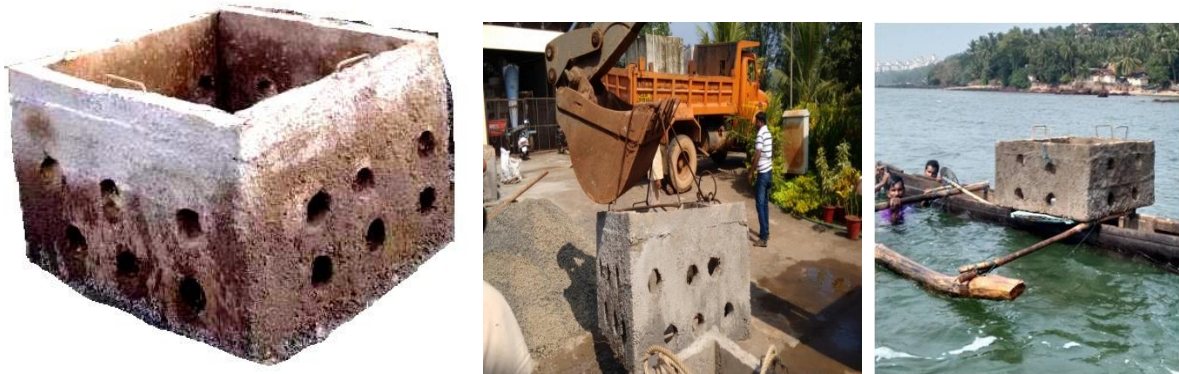
Fig.1 Construction and deployment of rectangular type AFHs
